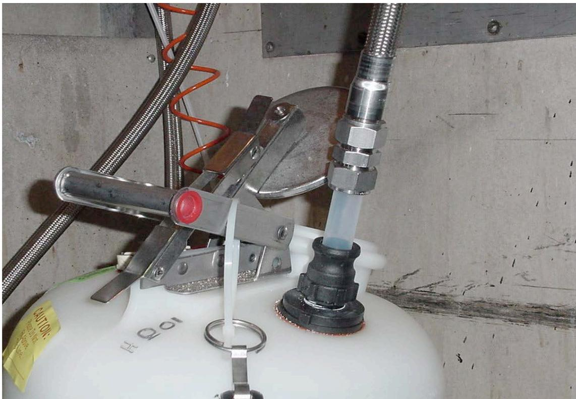
The pass through allows us to agitate the liquids in the container via a back flush circuit from the pump. This is used to clear any blockages in the tube or to cause the solids that have settled to go back into suspension. Both methods connect to the Xtractor, which pumps the waste liquids from the container to
